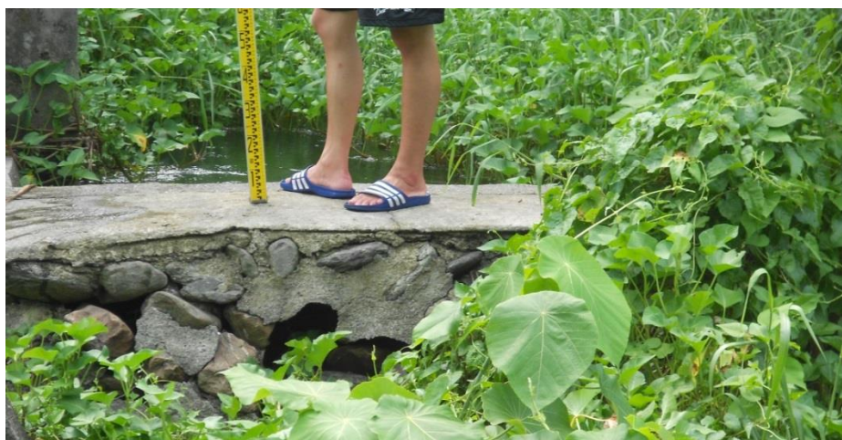
▲攔水堰已因常年失修而風化受損
