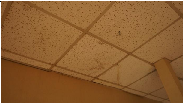
輕鋼架系統天花板汙損
